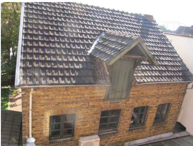
Westfassade in Backstein
